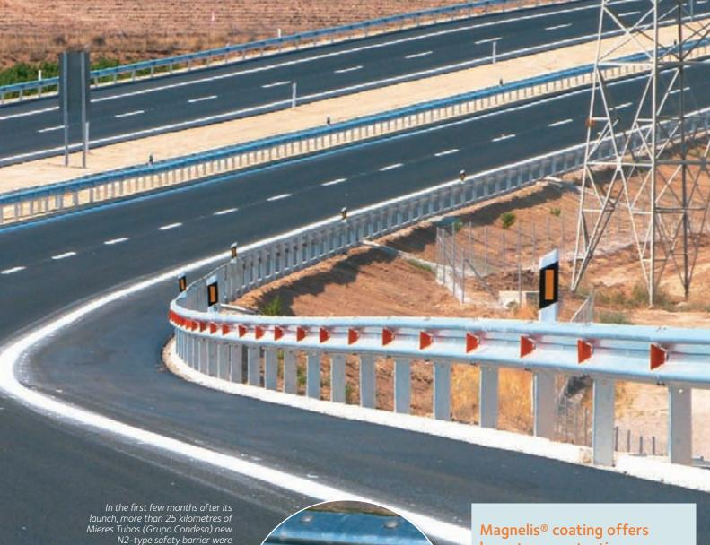
external certification body in the first quarter of 2012. The safety barrier now carries the CE marking, meaning that it meets the EN 1317 standard and can be utilised across Europe.
