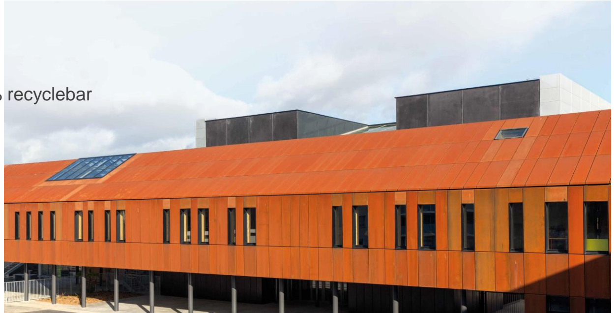
Educational and family center «Pôle Molière», Le Havre (France). ACAUM - Atelier BETTINGER DESPLANQUES Architectes associés. Picture © Paul Kozlowski
