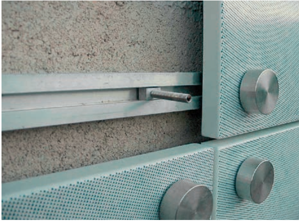
Fixing system for enamel panels (Signaux Girod, France)
